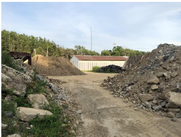
Stockpiles and rear of existing highway garage
